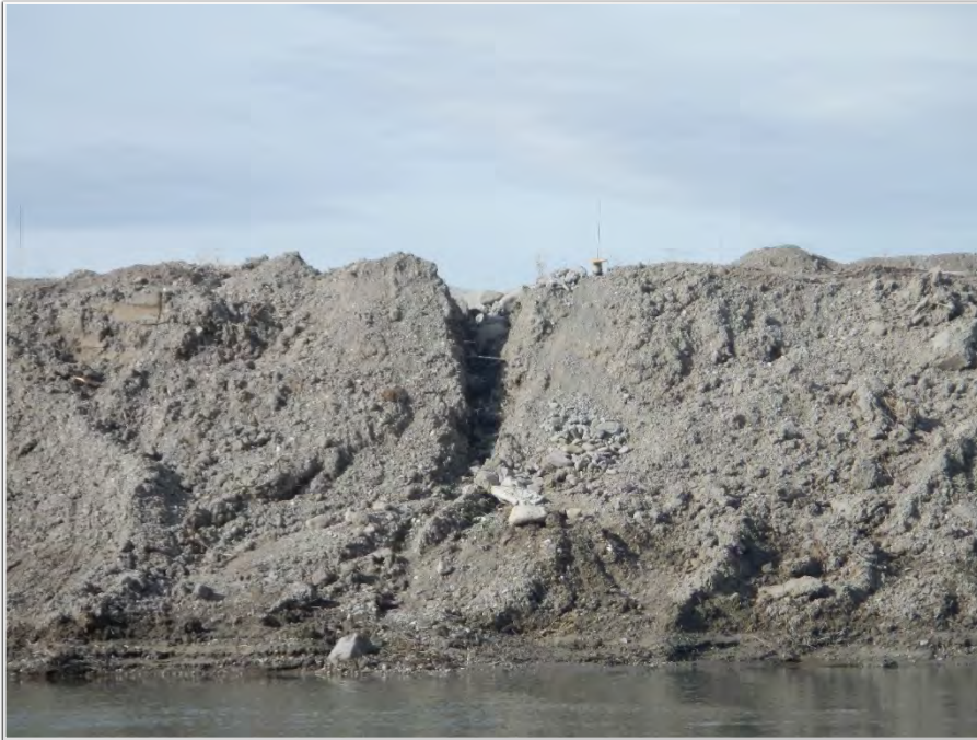
Figure 2.36. Poorly designed and cited land drain on sovereign lands.
