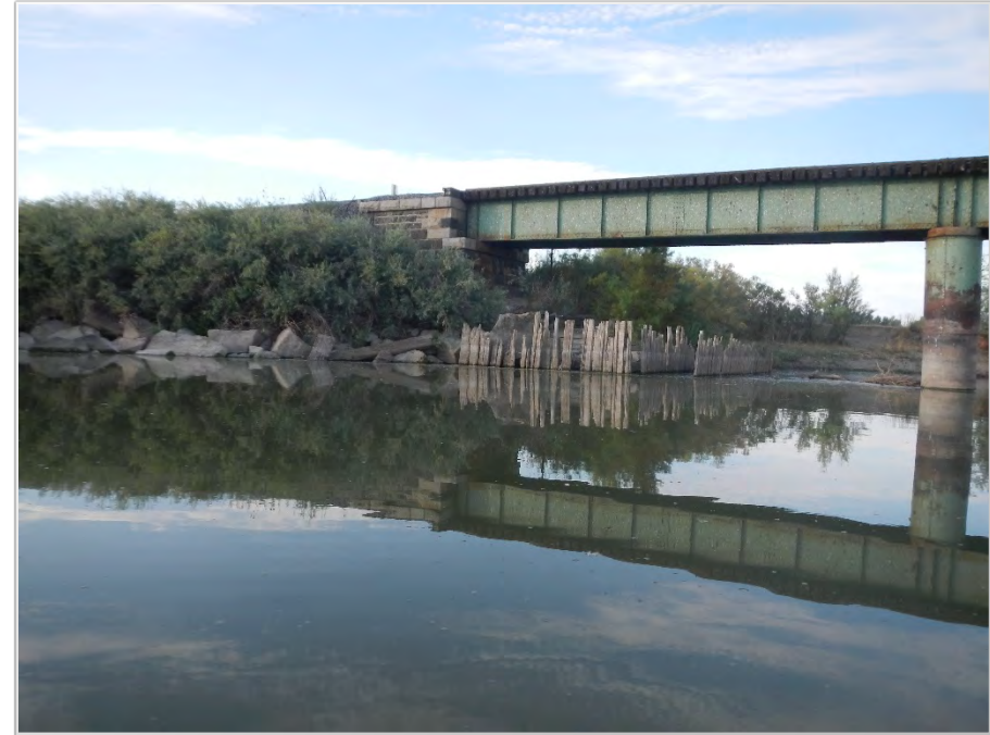
Figure 2.38. Above-grade crossing attached to a bridge on the Bear River.
